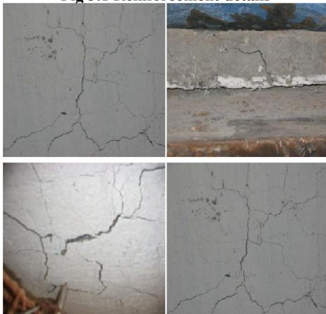
Fig 3.2 Crack Pattern in the Bottom Surface
